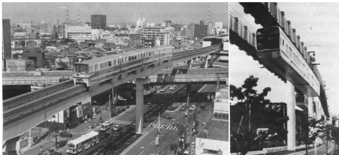
Figure 4 Two Different Type of Monorail. Straddle Form monorail, vehicle is supported on top of the rail (Left). Suspended Form monorail, vehicle is hooked below the rail (Right) (Shinya, 1988)
