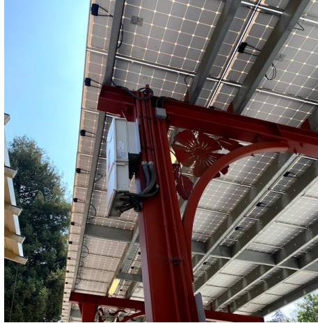
Figure 26 – Inverter and individual solar panel power optimizers mounted on structure. Location: Santa Cruz, CA.
