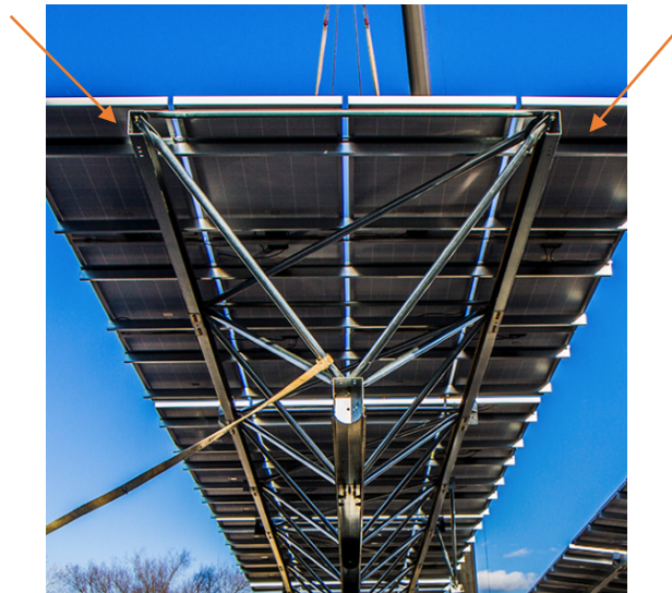
Figure 13: An underside view of Quest Renewables’ QuadPod Long Span Canopy design. Elements of this design can potentially be customized for the Superway since it satisfies a number of the installation challenges present (QuadPod Long Span Canopy, from (Quest Renewables, 2018))
