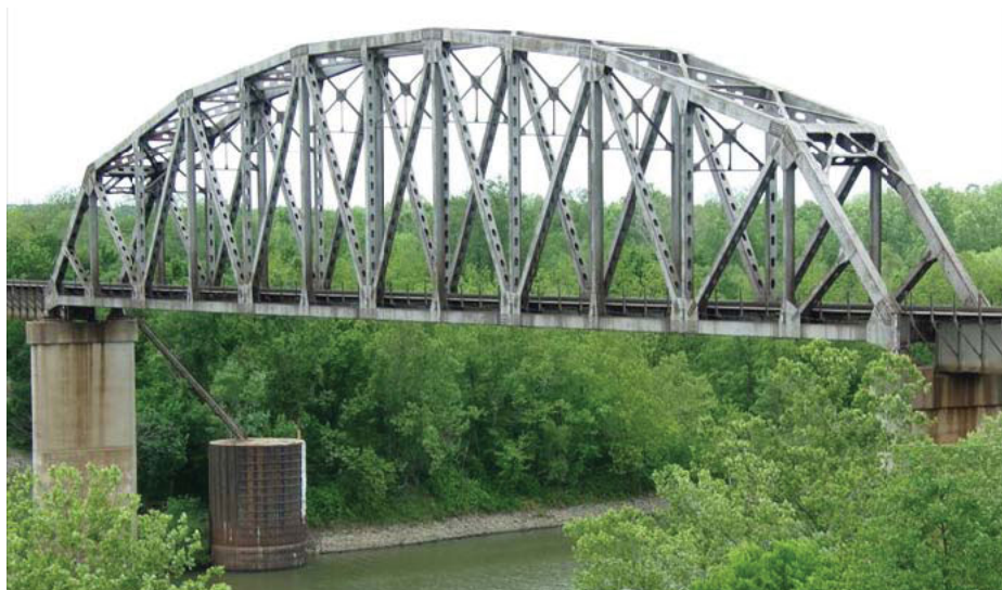
Figure 3. Polygonal Upper Chord. A polygonal upper chord on a Warren Truss with verticals used on a railroad bridge over the Verdigris River, Oklahoma (Steel Bridge for BNSF Railroad, from (Griggs, 2015)).
