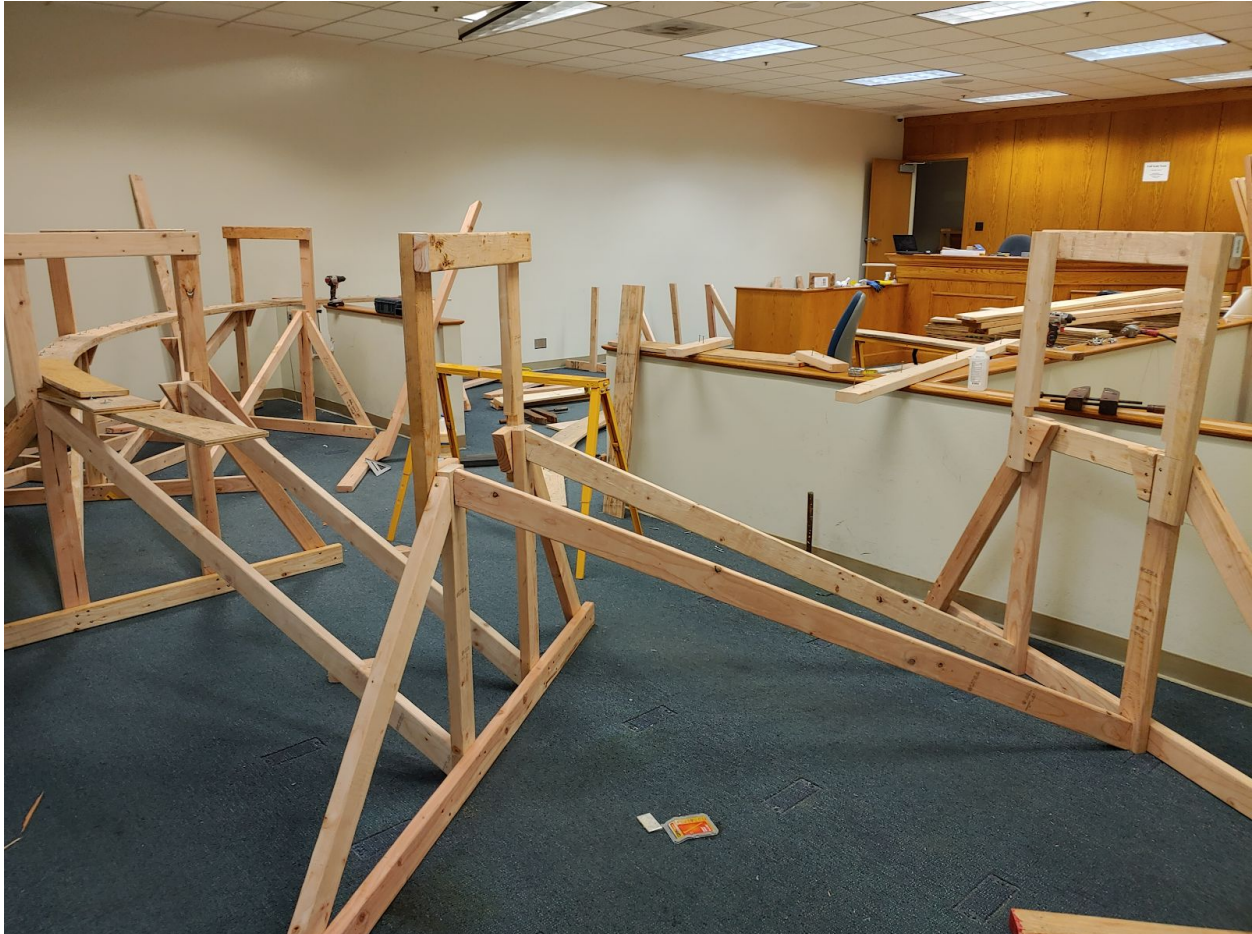
Figure 55: Actual uprights assembled with temporary lateral supports
