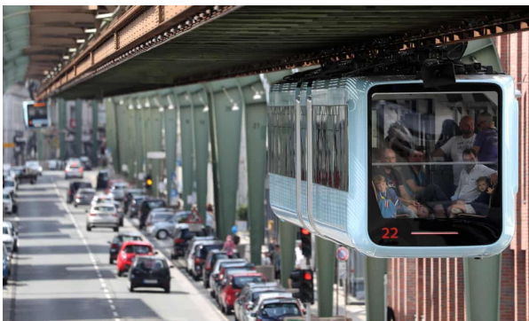
Figure 6. Wuppertal Suspended Railway above traffic.
