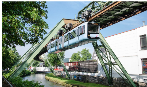
Figure 7. The Wuppertal Suspension Railway above the city river.
