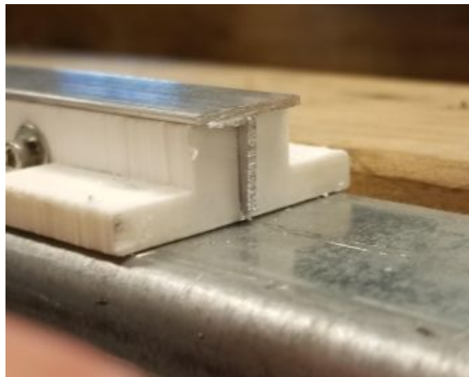
Figure 2. Existing aluminum rail and PLA insulated bracket
