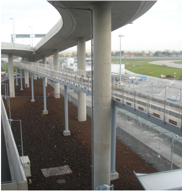
Guideway / Column Structure
