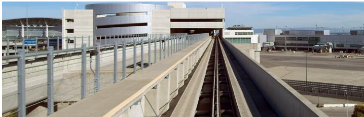
Figure 3: View of a Typical APM Guideway
