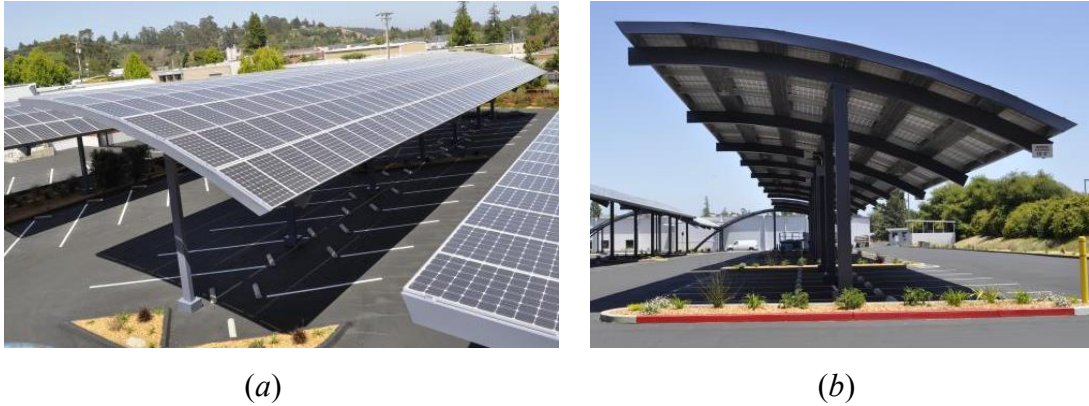
Figure 1—Example of a PV canopy installed over a parking lot. (a) is a top view to show the surfaces of the modules; (b) is a ground view to depict the supporting structure. Source: Swenson Solar [18]
