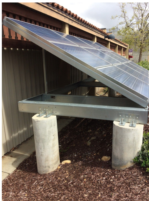
Figure 3. De Anza Solar Panel PV Rack.
