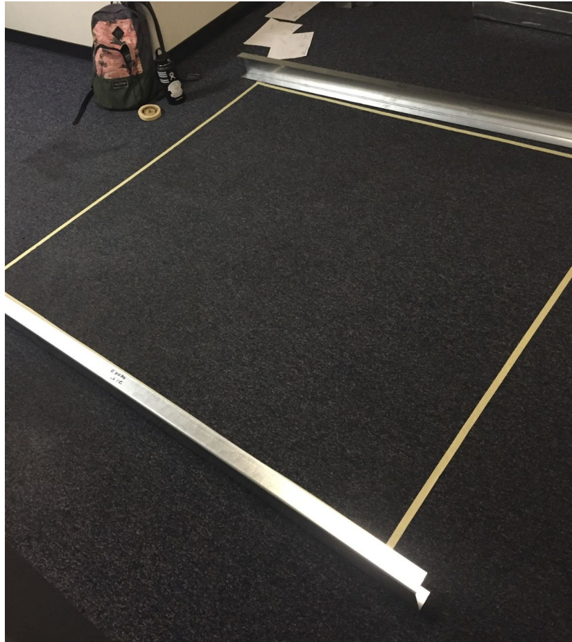
Figure 46. Process of laying out purlins for base frame.
