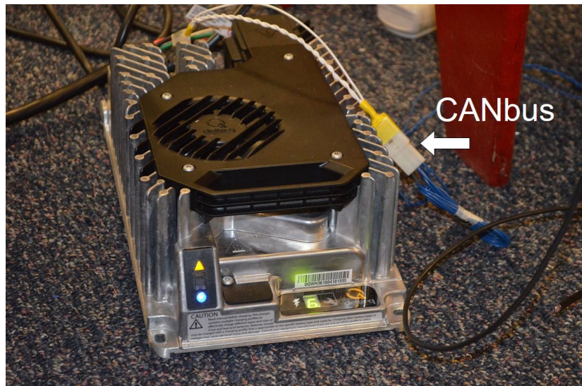
Figure 23: Delta-Q IC 1200W Charger and the CANbus communication quick plug-in port as the charger is not located on the bogie (off-board). Each time the bogie needs to be charged, this connection must be physically made.
