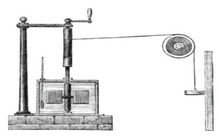
■ Fig. 14.2 Lavoisier's experimental approach to measuring the oxygen content of the atmosphere (Source: Florida Center for Instructional Technology)
