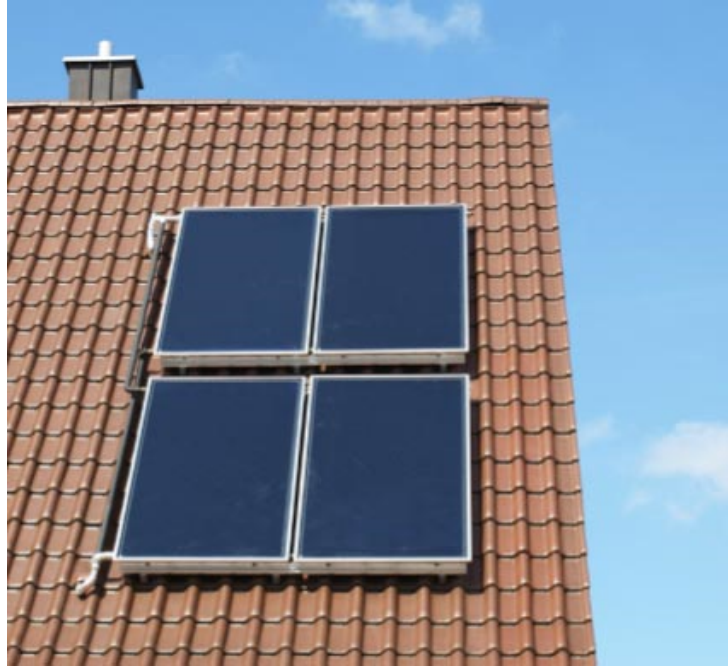
FIGURE 1.20: Solar thermal flat plate collector.
