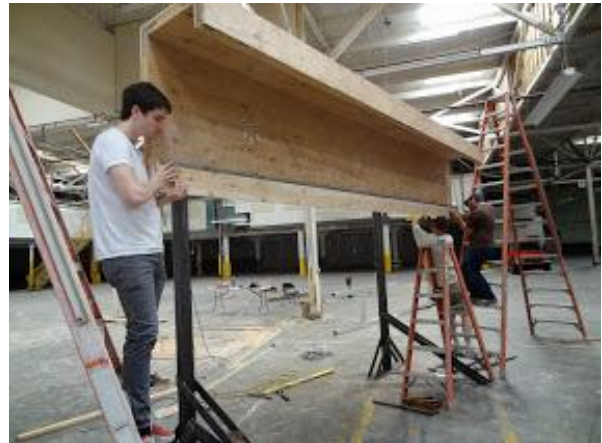
Figure 23 Initial Bolting of Guide Way to Support Columns.
