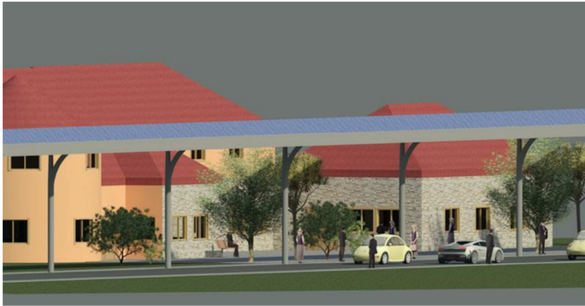
Figure 86. Representation of the integration of the structure into a city environment. This virtual image depicts the aesthetics of the structure of the guide ways and columns, which minimizes the visual impact due to the height of the structure and the slim columns.
