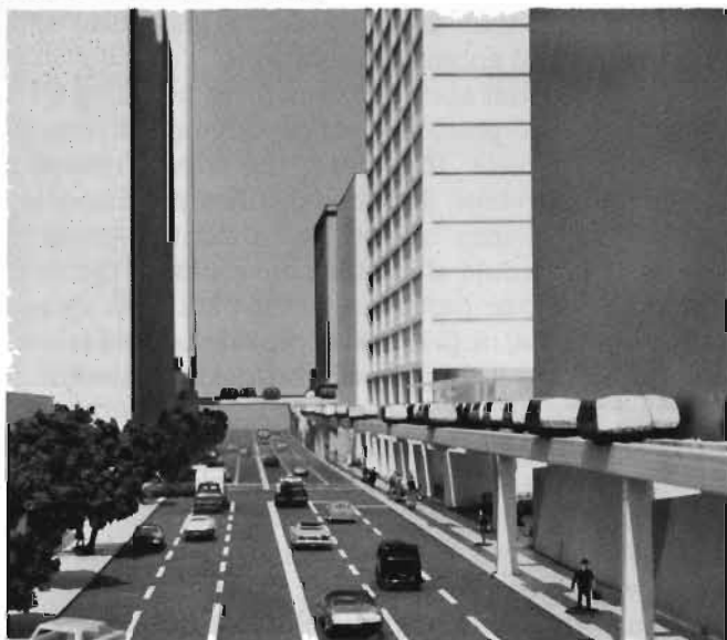
Fig. 2-5. Typical Curb-line Alignment for One-Way PRT
