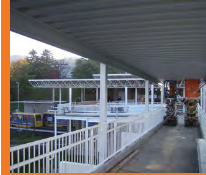
An intermodal facility was added last year to one of Morgantown's stations
