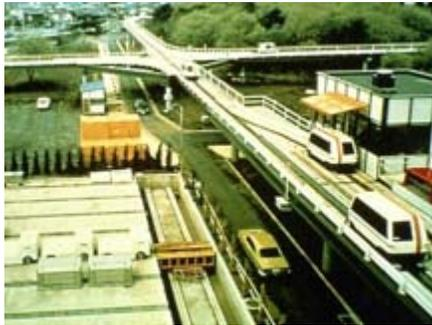
**CVS.** The Computer-Controlled Vehicle System (CVS) is a one-second-headway, 2000-lb, four-passenger-vehicle PRT system developed in Japan beginning in 1968. Scale models were built, a 1000-vehicle network was simulated, and a full-scale test facility began operating in 1972 in a suburb of Tokyo with 4.8 km of guideway and 60 vehicles. Extensive
